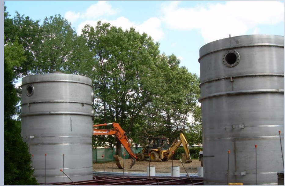
Air Strippers being installed at Well Nos. 1 & 2
