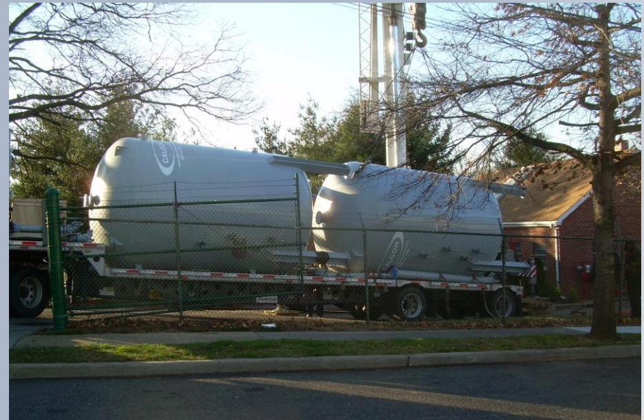
GAC being installed at Well Nos. 4 & 5
