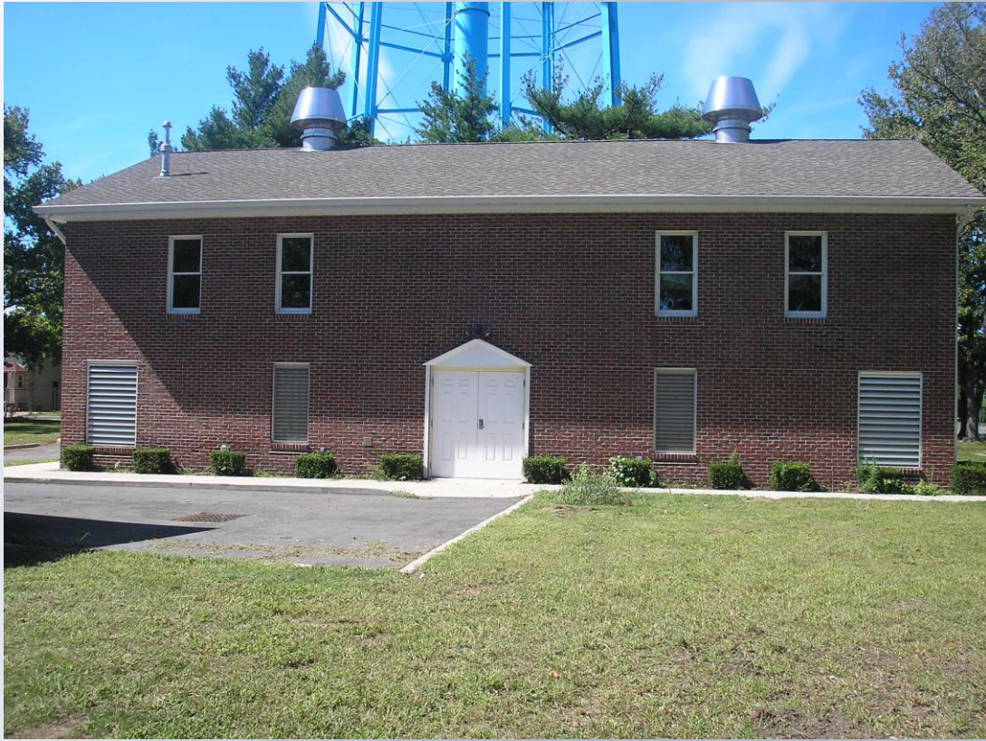
Air Stripping Facility at Well Nos. 1 & 2 - Schroeter Avenue
